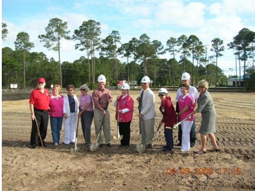
Groundbreaking for the new Panama City Beach Public Library at 12500 Hutchison Blvd.
