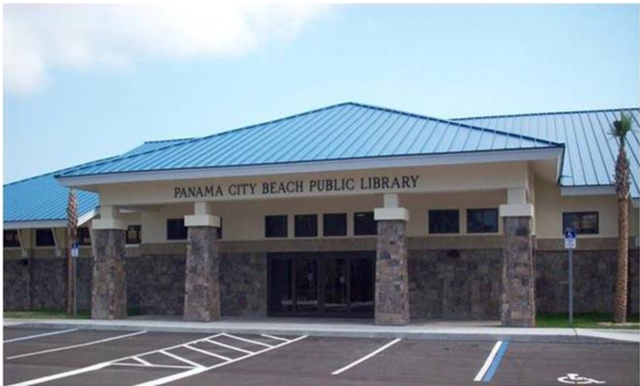
Panama City Beach Public Library building at 12500 Hutchison Blvd.
